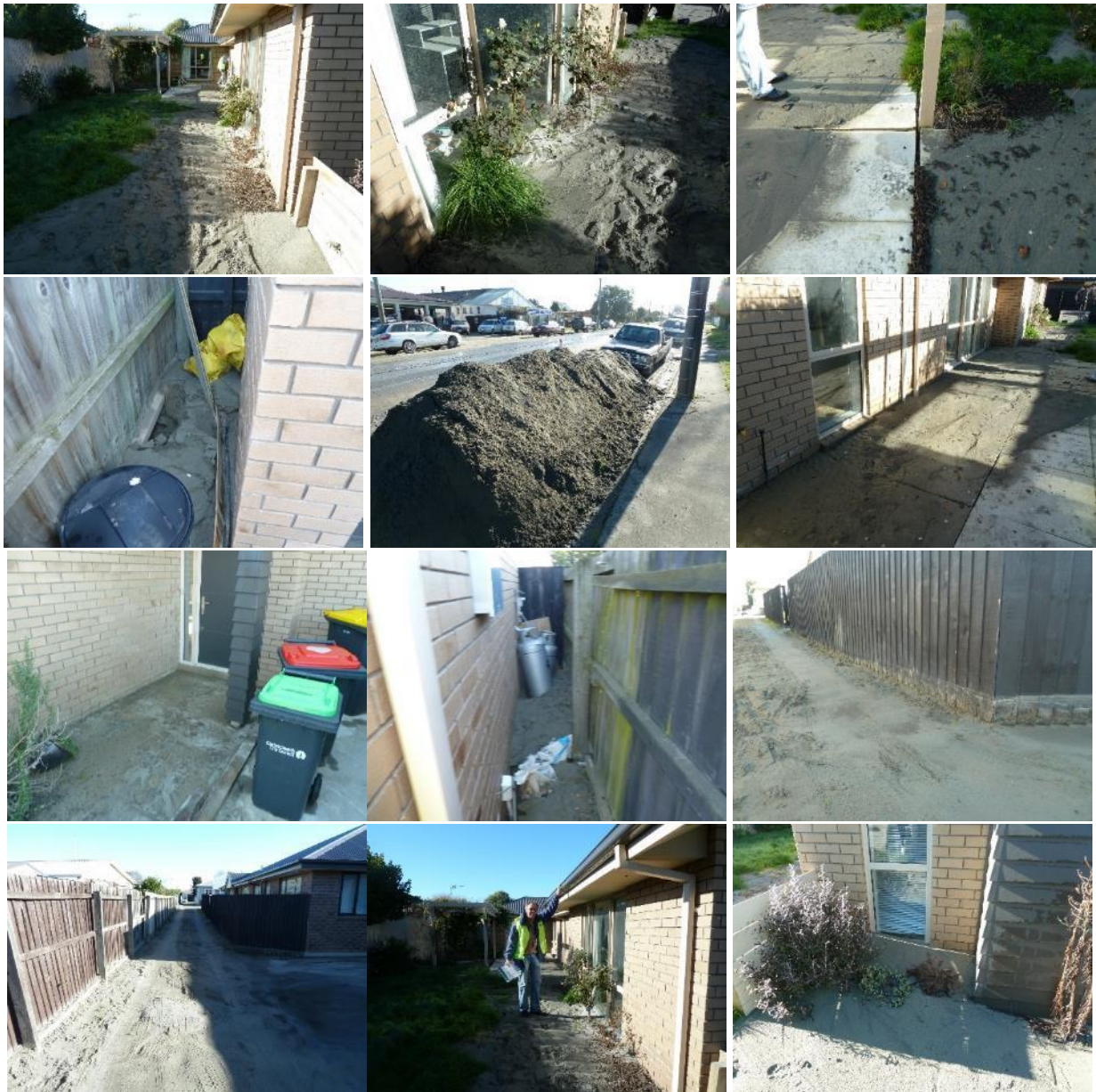
Figure 78: Ground photographs showing the property with Patch C and ejecta remnants within Patch C (photograph date: July 2011). The ground underwent lateral spreading.
